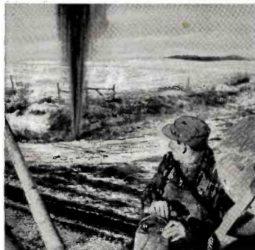
MINIATURE EARTHQUAKES like this were set off by the hundreds of thousands last year to chart underground rock formations, permitting exploration crews to pinpoint likely oil drilling locations. Even using latest scientific equipment, odds against finding new oil are great.
